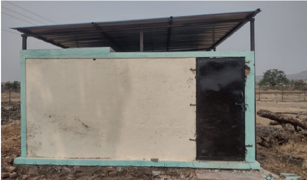
Toilets renovation work done in high school
